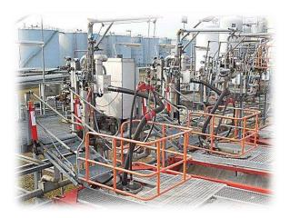
Isopad can offer Flexible Transfer Lines with approved trace heating systems for use in hazardous areas along with integrated sensor technology for intrinsic safe circuits. Following technical design guidelines the transfer lines as well as all exposed parts to the explosive media or ambient conditions are being conductive to reach a maximum on personal and product safety.
