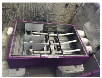
Fitted with ceramic pillars, side plates and phase separators. Clad with K-Mass™
