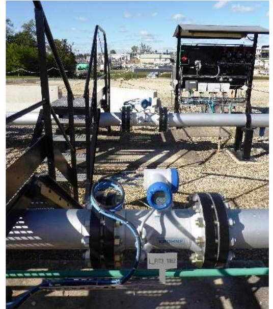
OPTISONIC 7300 ultrasonic flowmeter measuring natural gas
