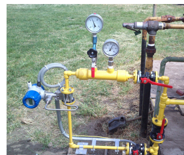
Installation of flowmeter with sandwich connection
